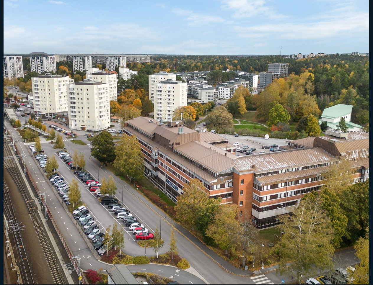
Ongoing tenant adaptation for Region Stockholm, 3 000 sq.m in Täby - Stockholm
