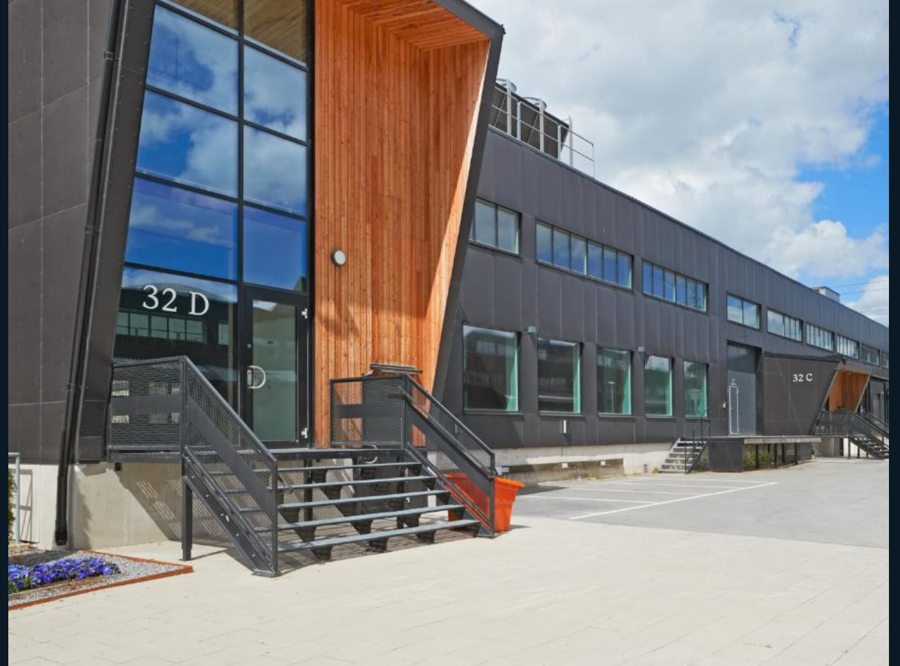
Ongoing tenant adaptation for Smartoptics, 4 178 sq.m in Kista - Stockholm
