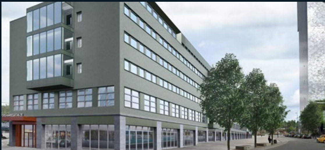
STOCKHOLM Kista, Helgafjäll 1 Tenant adaptation completed, Mycronic
