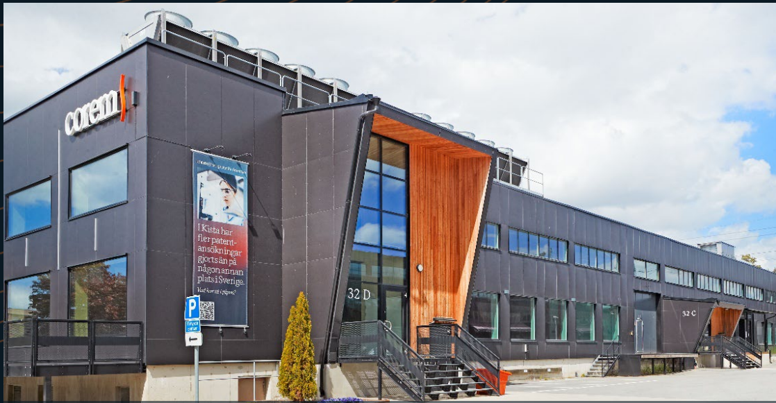
STOCKHOLM, Kista Ongoing tenant adaptation for Smartoptics, 4 178 sq.m
