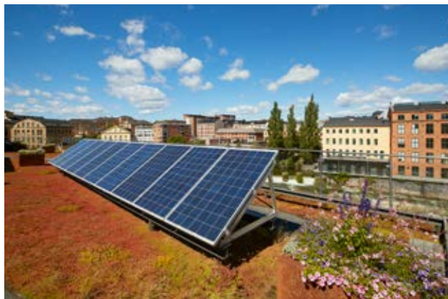
Sedum roof and solar panels in Norrköping.
