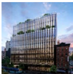
PARK VIEW (118 10TH AVE), NEW YORK, KONTOR
